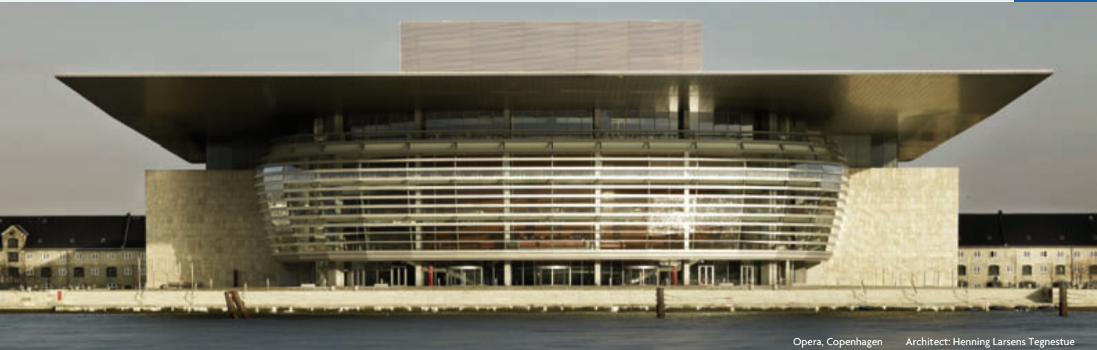
Opera, Copenhagen Architect: Henning Larsens Tegnestue
